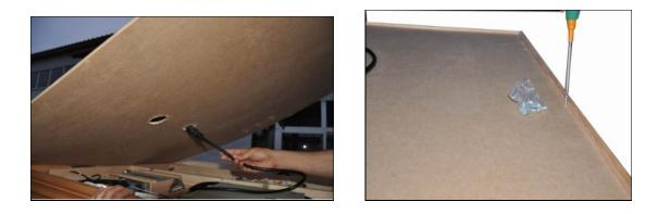
**Step Ten**: Return to the Installation Bolts on the Left and Right Panels. Using a screwdriver tighten the bolts as necessary.
