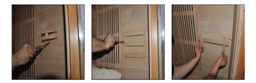
**Step Twelve:** Install the Ionizer (this step is optional if you have the Cedar Wood option, as Cedar is naturally anti-bacterial). When you look inside your sauna, you will see a black wire hanging down from the top left side of the ceiling. Screw the Ionizer vertically below the wire, as seen in the picture below. Note that the disk on the back of the Ionizer can stay in the "on" position. Refer to "how-to-use" instructions on page 21 for operation.
