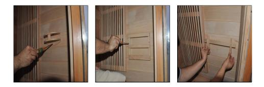
**Step Thirteen:** Install the Ionizer (this step is optional if you have the Cedar Wood option, as Cedar is naturally anti-bacterial). When you look inside your sauna, you will see a black wire hanging down from the top left side of the ceiling. Screw the Ionizer vertically below the wire, as seen in the picture below. Note that the disk on the back of the Ionizer can stay in the "on" position. Refer to "how-to-use" instructions on page 21 for operation.
