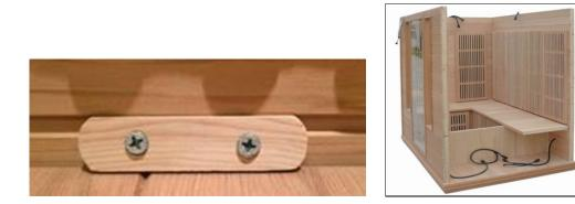
**Step Six**: From Box B, install the Right Panel by lining up the panel to the Front and Back Panels. Using the Installation Bolts provided in the accessories box, thread the Bolts through the holes in the Right Panel to the Front and Back Panels. Finger tighten the bolts. A final tightening of the Bolts will be performed with a
