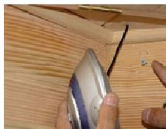
**Please note that you can adjust glass door. First, loosen the screws that attach to hinges. Second, adjust glass door. Third, re-tighten the screws.**
