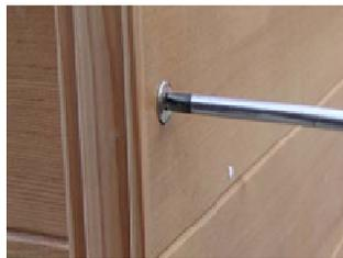
**When all panels are in place tighten all screws to fully secure Sauna**
