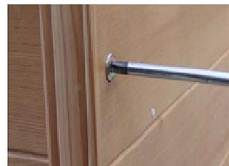
**When all 4 panels are in place tighten all screws to fully secure Sauna**
